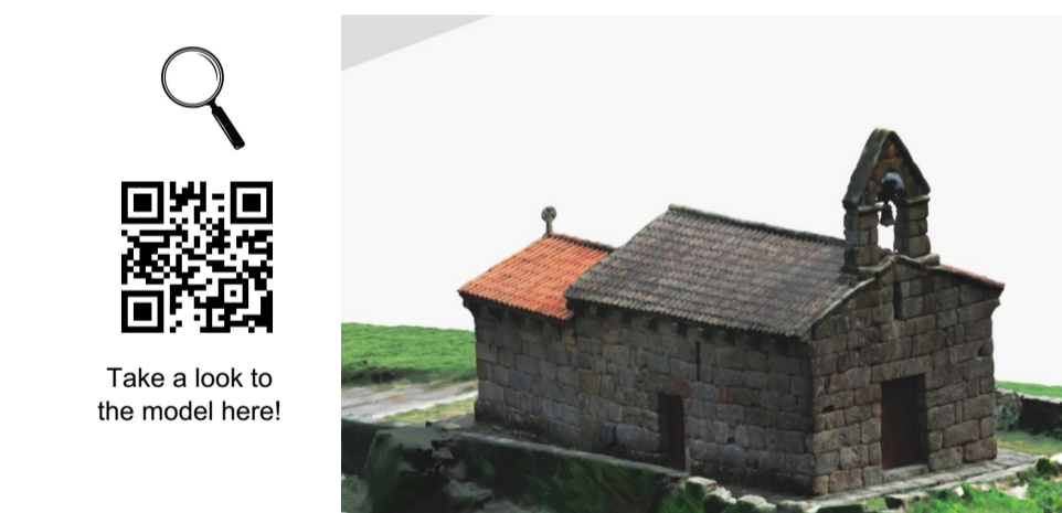
Figure 2: Picture of the North-West elevation of the Church
